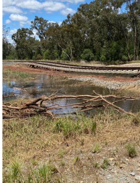
Plate C7.19 – Collapsed section of railway immediately to the east of Overland Road.
