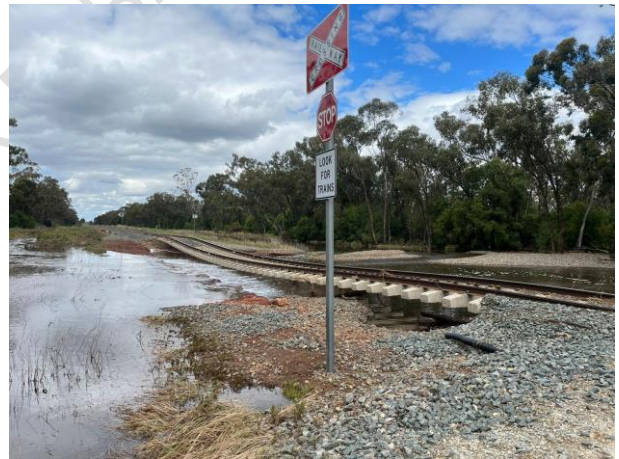
Plate C7.19 – Collapsed section of railway immediately to the east of Overland Road.
