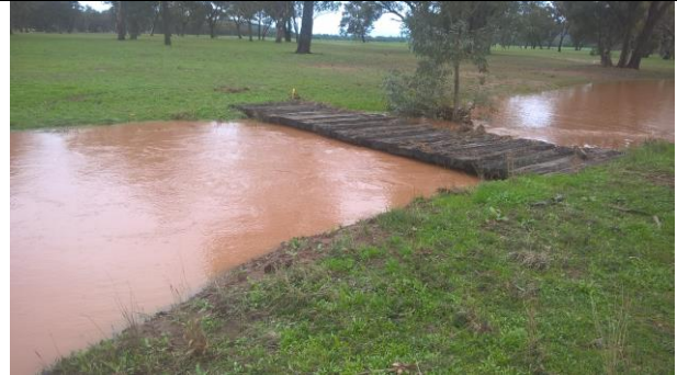
Plate C4.2 – Flooding in the vicinity of the old bridge adjacent to the 4 th fairway of the Bogan Gate Golf Club.
