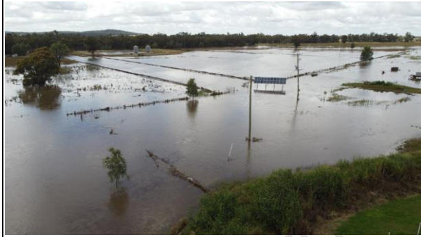
Plate C7.14 – Flooding in the vicinity of the Myalls homestead.
