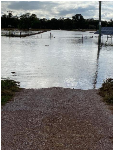
Plate C7.7 – Flooding in the vicinity of the Myalls homestead.
