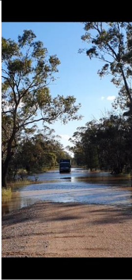
Plate C6.7 – Floodwater inundating the Tubby Lees Road causeway crossing of Gunningbland Creek.
