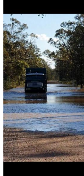
Plate C6.8 – Floodwater inundating the Tubby Lees Road causeway crossing of Gunningbland Creek.
