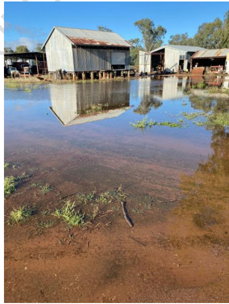
Plate C7.4 – Flooding in the vicinity of the Myalls homestead.
